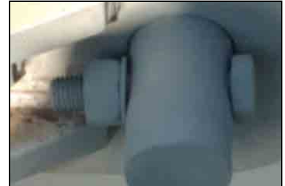
The pins were successfully restored and protected from further corrosion.
